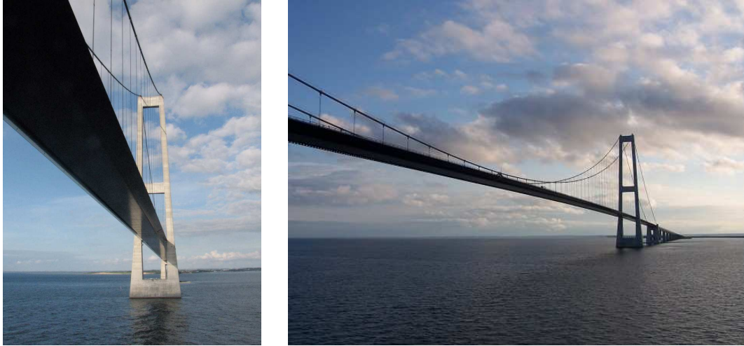
Figure 3.3: Great Belt East suspension bridge.
