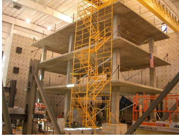
Figure 1: Overall view of the full-scale 3-story flat-plate building test specimen.
