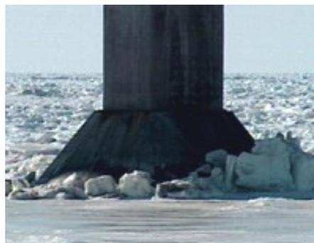
Figure 3. Ice impacting with pier, Confederation bridge
