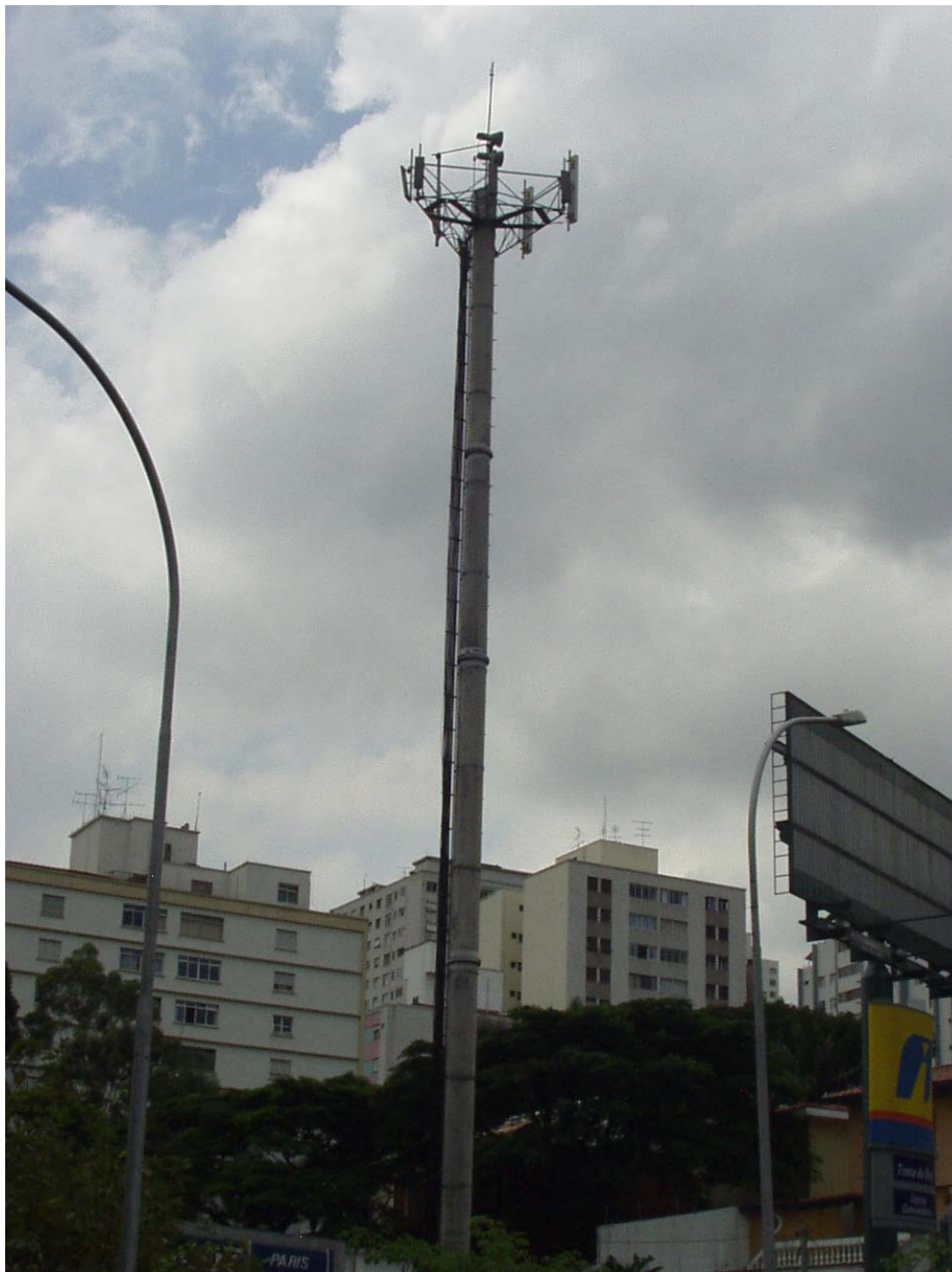
Fig. 1 – Typical pre-cast RC telecommunication tower
