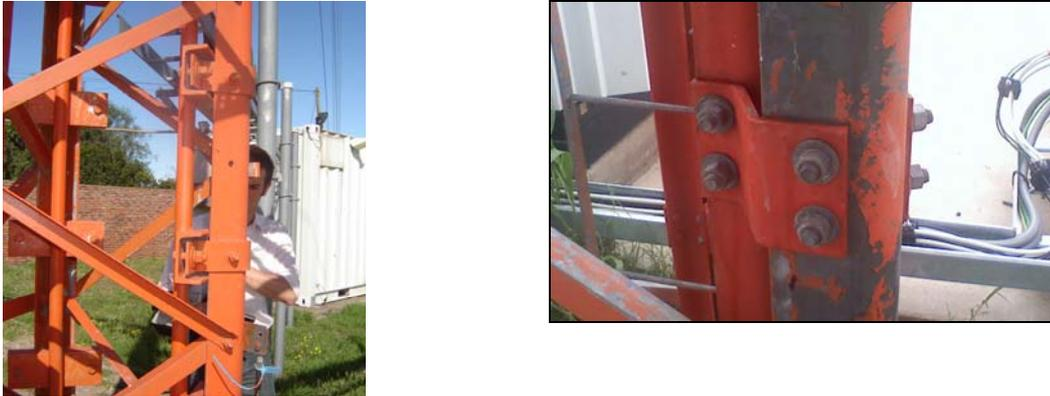
Figure 1. Examples of joints for a reinforced tower.
