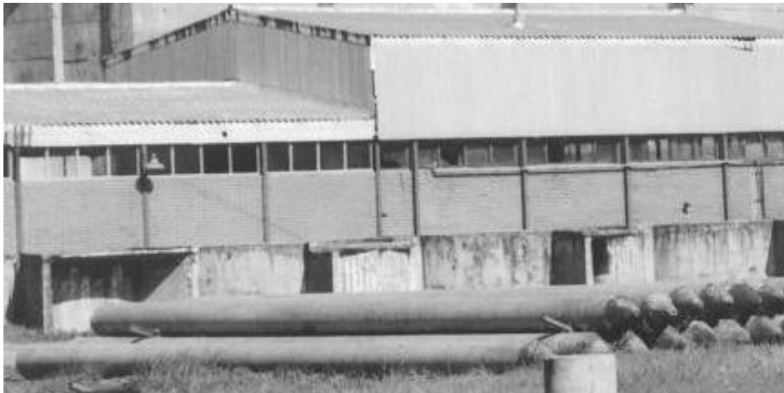
Figure 3. Concrete annular piles tested in CTNOA S.A.
